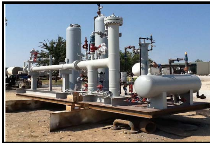
Figure 2. Photograph of the Membrane system at Marathon Oil drilling rig facility in Texas.
