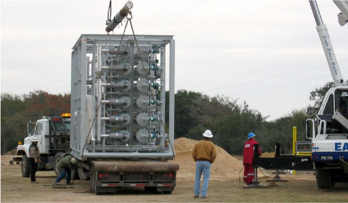
**Figure 5. A standard membrane-based CO<sub>2</sub> treatment unit is lifted from the truck.**
