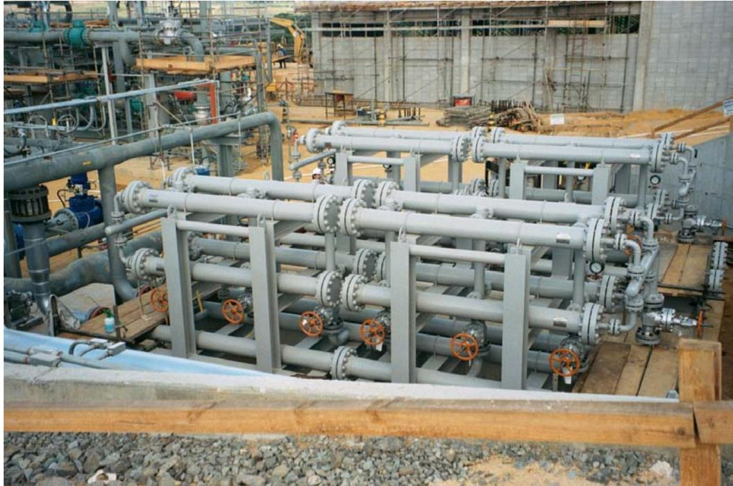
**Figure 3. A typical membrane skid; sixteen carbon steel pressure tubes house the membrane modules.**
