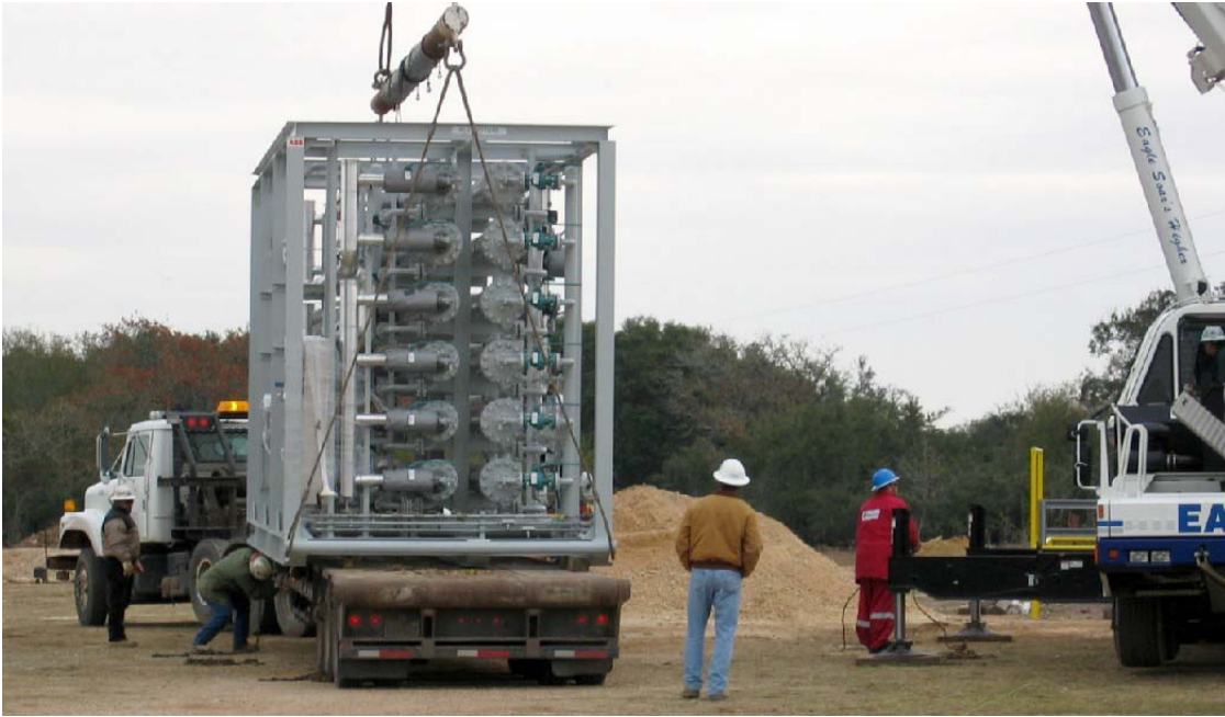
Figure 5. A standard membrane-based CO 2 treatment unit is lifted from the truck.
