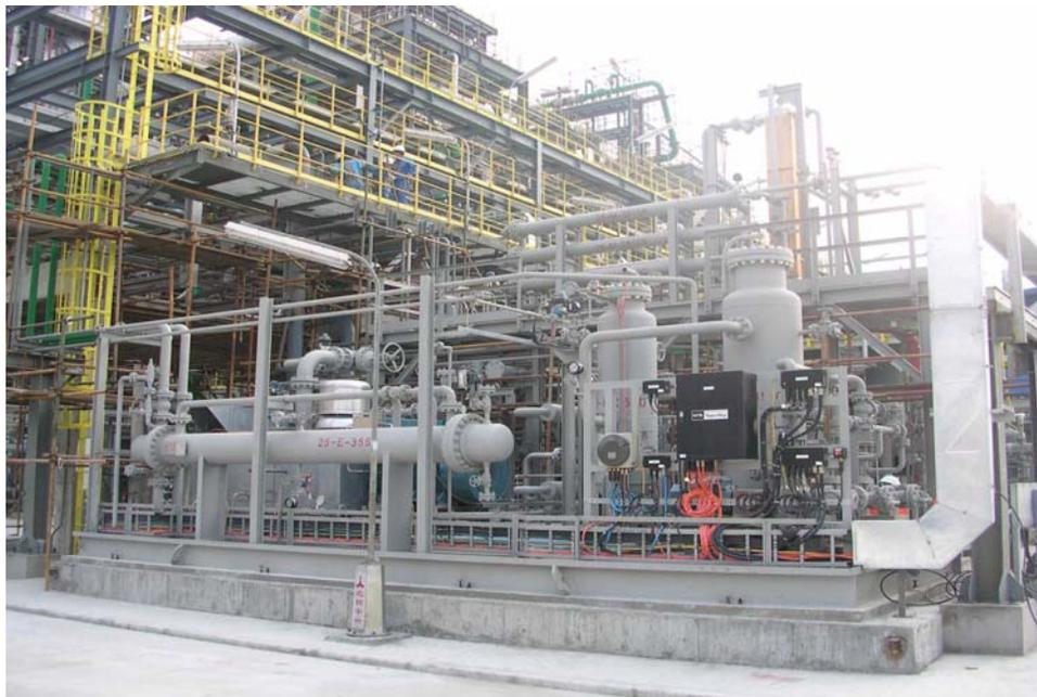
Figure 7. Photograph and process flow diagram of a membrane propylene recovery system installed at a modern polypropylene plant. The front portion of the unit is the compressor package. The spiral-wound membrane modules are contained in the horizontal tubes above and behind the compressor. This unit recovers approximately 1,000 lb/h of hydrocarbons.
